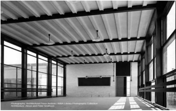
Figure 1. Clear exhibition of structural components in Hunstanton School (Source: RIBA Library Photography Collection)
